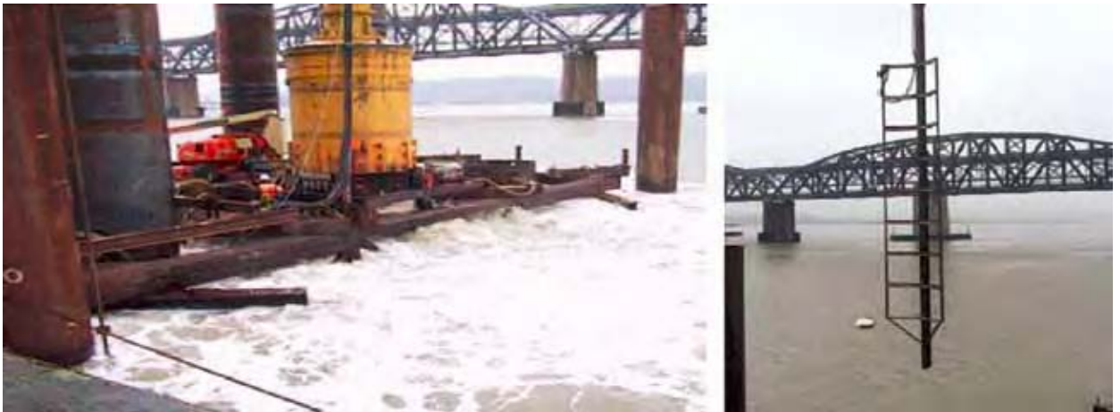
Figure 2.20 Multiple-stage unconfined bubble screen system (CALTRAN 2009)
